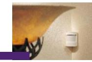
identify body heat to detect intruders. They're adjustable so pets can move about freely.
